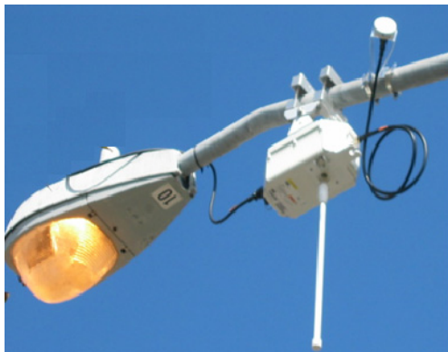
Figure 8-3 1500 Series Mesh AP Installation
